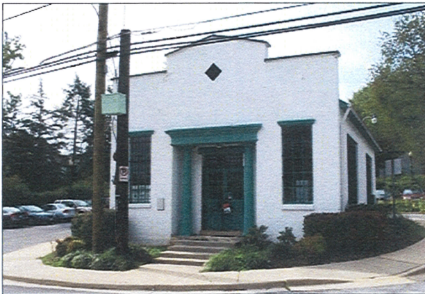
Germantown Bank, 1922, brick structure 19330 Mateny Hill Road
